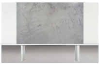
FULL SLAB VIEW
