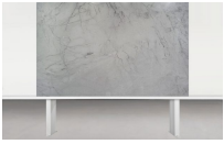
FULL SLAB VIEW
